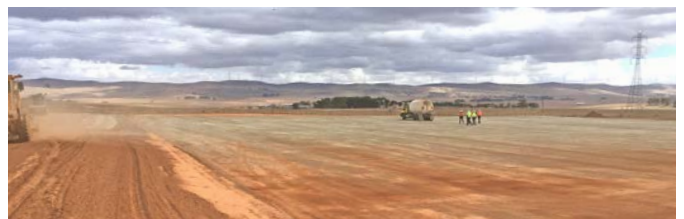
Substation works as at 30 March, 2017.
