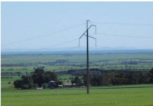
Figure: An example of a 132kV power line pole used in SA to transmit electricity from a wind farm to the transmission line.
