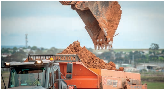
Above: Heavy equipment places topsoil over the clay, ready for grass seeding.
