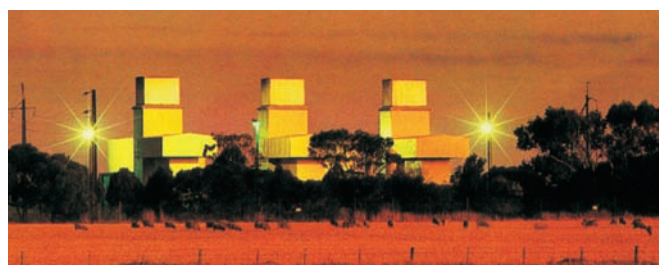
Snuggery power station
