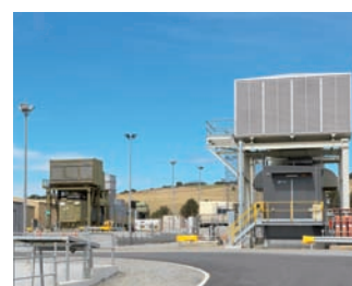
Port Lincoln power station
