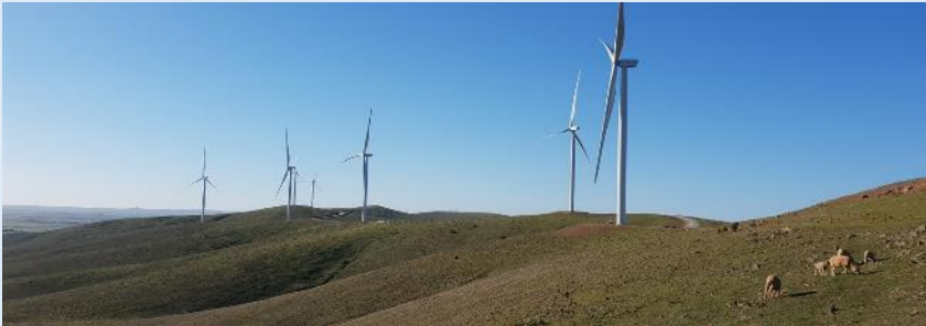
Willogoleche Wind Farm, SA (119MW); completed construction in 2019
