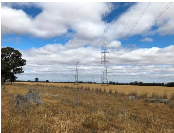
Plate 13 Transmission powerline easement (facing north-west)
