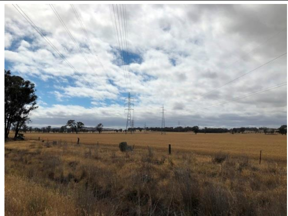
Plate 14 Transmission powerline easement (facing south-east)
