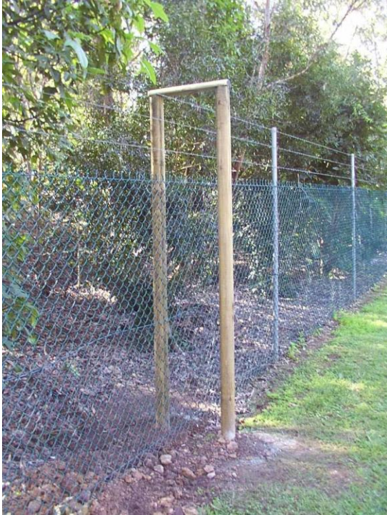
Plate 2 Example of fauna friendly security fence that could be adapted for the climbing fauna species.
