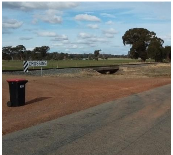
Figure 3-4 Goorambat-Chesney Road and Spinks Lane intersection
