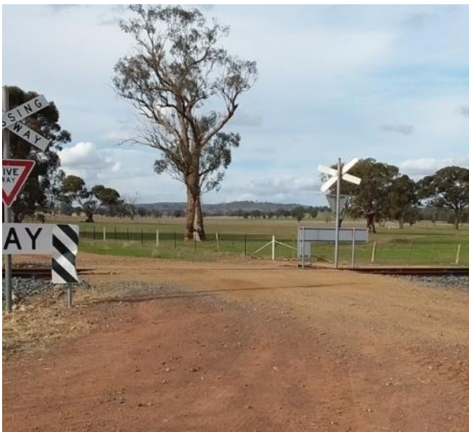
Figure 3-3 Level-crossing on Spinks Lane
