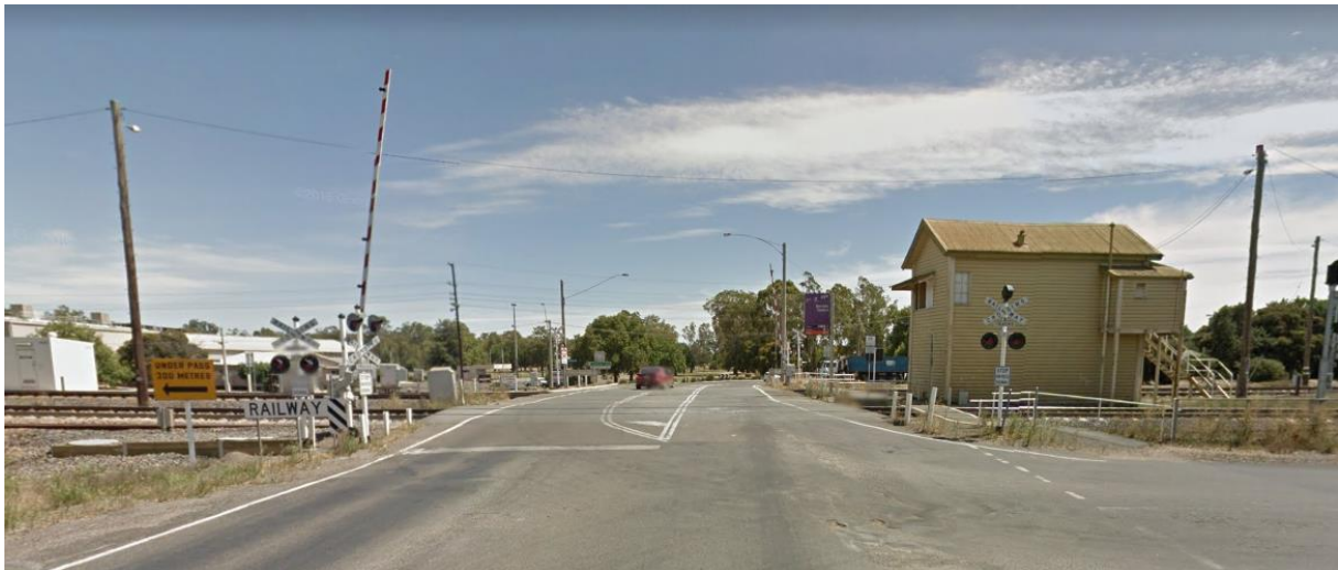
Figure 11 Active protection level crossing on Midland Highway in Benalla
