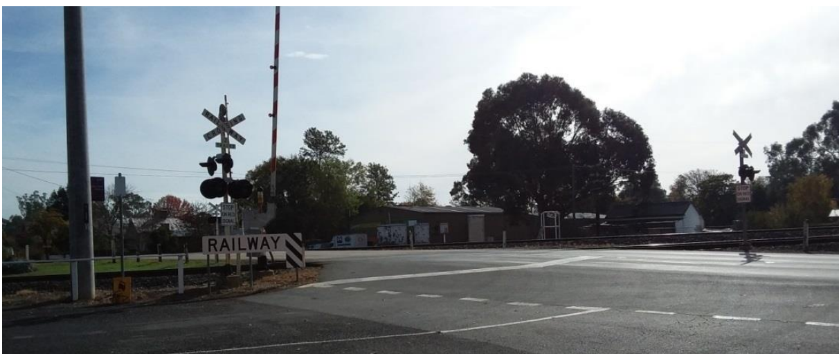
Figure 10 Active protection level-crossing intersecting with Nunn Street in Violet Town
