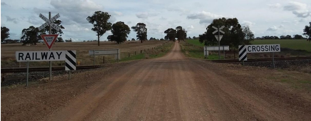
Figure 6 Peck Road intersecting with rail level crossing
